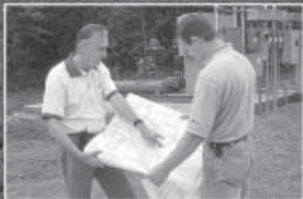
Professional Irrigation System Repairs, Renovations, New Construction
